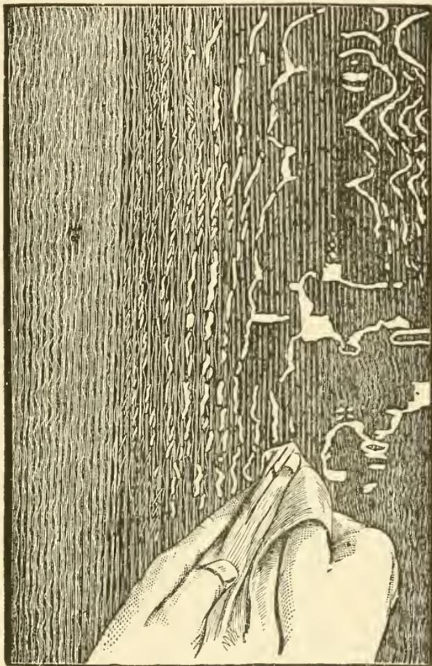
Fig. 32. Wiping Out Figure in Oak Graining.
